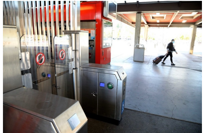
A new, harder-to-evade style of faregate shown at Concord Station, part of parallel “station hardening” efforts for greater safety and security
