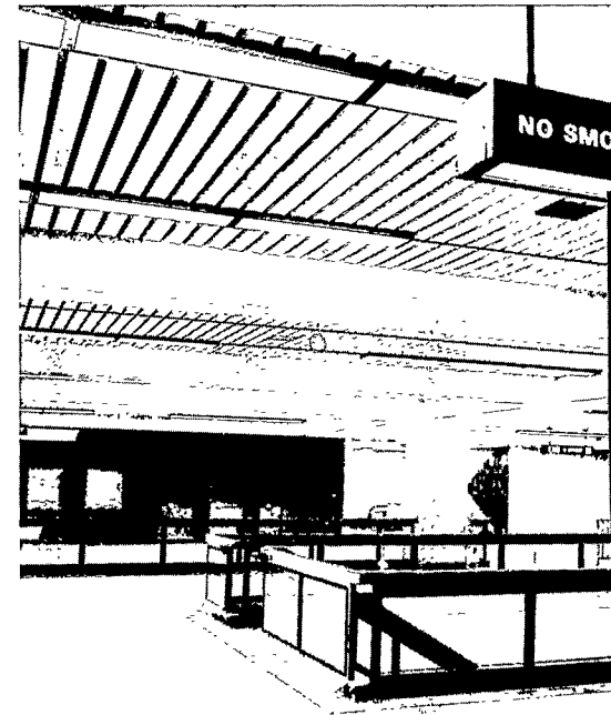
Mezzanine—Lake Merritt Station
