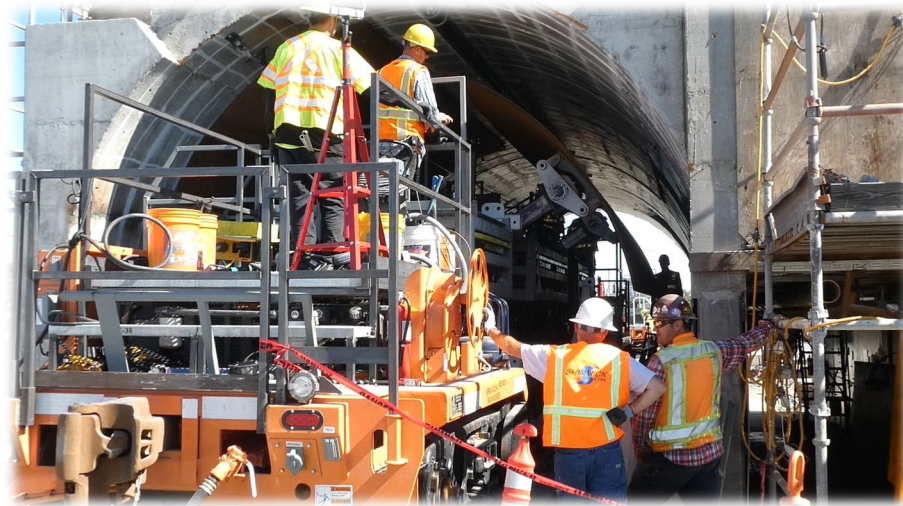
Tube Mockup for Retrofit Bore Installation
