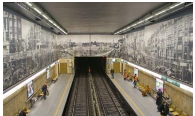
LED lighting upgrade at a station in Brussels, Belgium has reduced energy consumption by half Source: http://www.schreder.com
