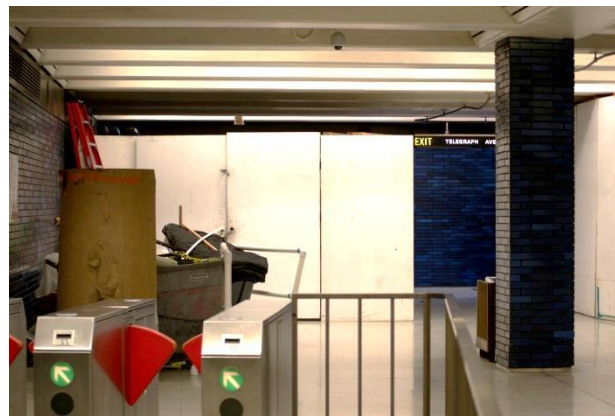
Figure 20: Maintenance Equipment Stored in Public View
